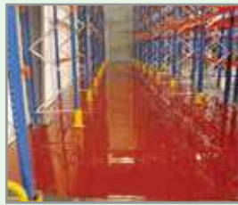
Racking Sections (Warehouses)
