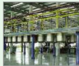
Minimum Downtime for Production (Production, Food Mfg, F&B Plants, High Tech Mfg)
