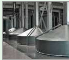
Cold Storage (Production, Dairies, Food Mfg, Plant Rooms, F&B Plants)
